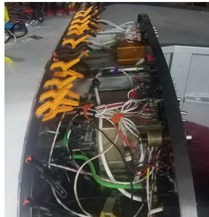
Mini-clamps holding the seal in place during curing
